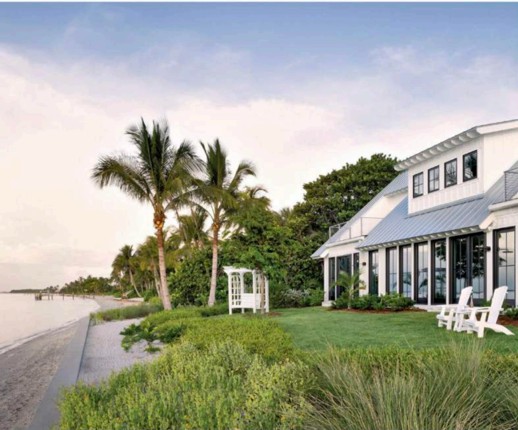
Above: At the back of the property, landscape designer Robert S. Walsh provided erosion control by installing golden creeper, spartina and mully grasses, sea oxeie daisy, and lowgrass to create a native buffer that blends in with the waterline. Merida offered a spot to enjoy the view using chairs and a side table by The Best Adirondack Chair Company.
